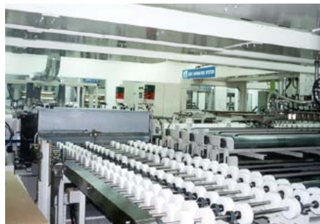
Entrance to Scrubber
