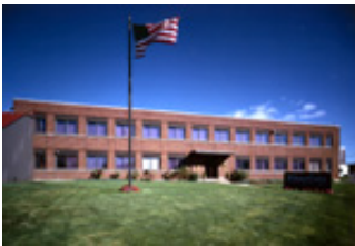
FiberCote Industries Waterbury, CT
